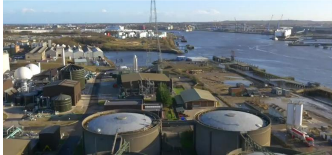
Figure 1 – Aerial Photograph of sludge processing area of Tyneside Wastewater Treatment Facility, Newcastle
